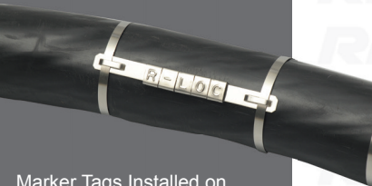
Marker Tags Installed on Power Cable
