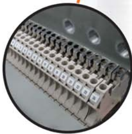
Terminals in connection box for load circuits
