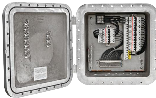
w/o main breaker
